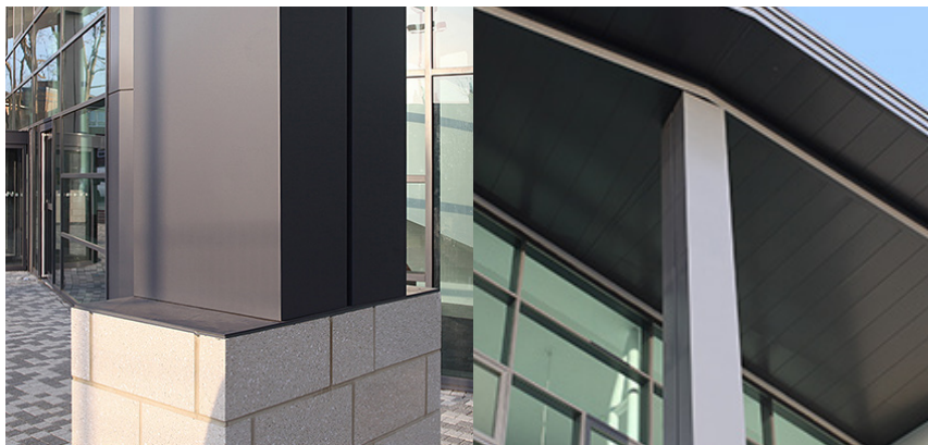
Powder coated aluminium column casings
